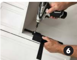
Drill top hinge holes
