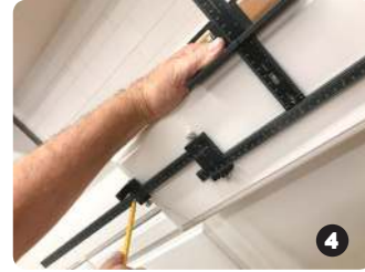
4 Set small end stop to half the drawer width
