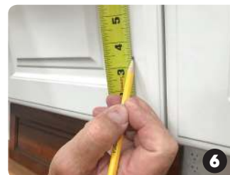
We are setting this one 3 1/2" from the bottom
