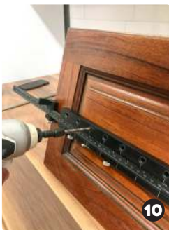
9 Hold stops firm against top and left side of drawer and drill your holes
