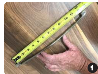
Measure hardware hole spacing
