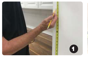
Measure and mark desired location
