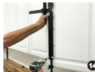
Holding side and bottom stops against door drill bottom hole
