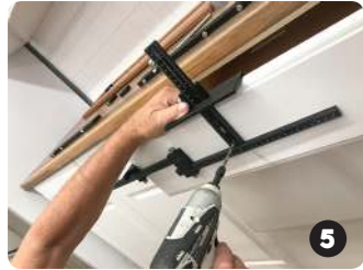
5 Now you are ready to drill an entire drawer bank
