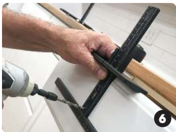
Drill hole using fixed center drill bushing
