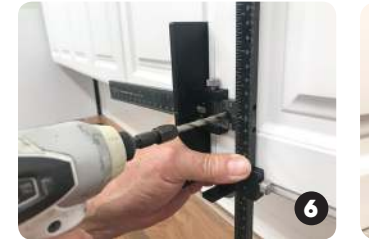
6 Position tool with stops as shown and drill hole through drill bushing
