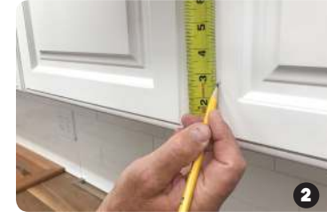
2 Measure from bottom mark position with pencil
