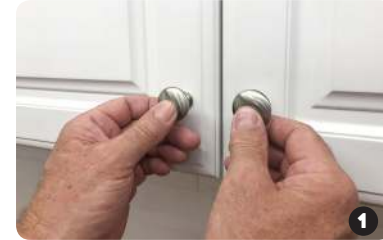
1 Place hardware to find the position you like
