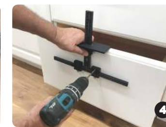
Center on drawer and drill holes
