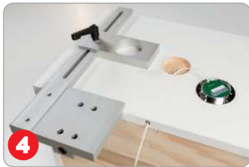
4 Remove clamps and feed wire through by hand
