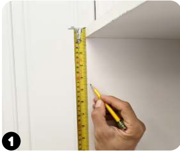
1 Mark center of hinge plate.
