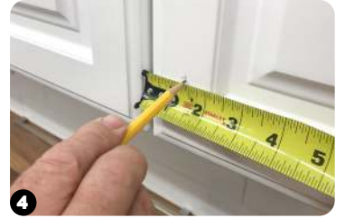
4 Measure from side of door to mark.
