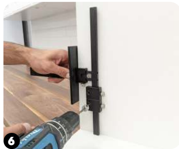
6 Flip tool to bottom of cabinet, position tool with Large Stop and T-Square firmly against cabinet surface, and drill second set of holes.
