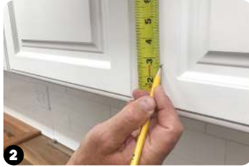
2 Measure from bottom of door to mark.
