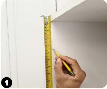
1 Mark center of hinge plate.
