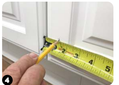
4 Measure from side of door to mark.
