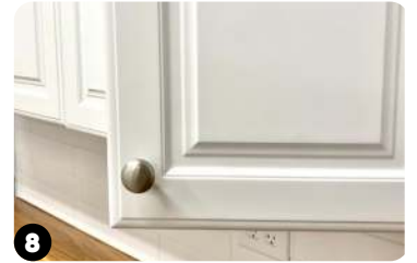
8 Install knob and repeat process for additional doors.
